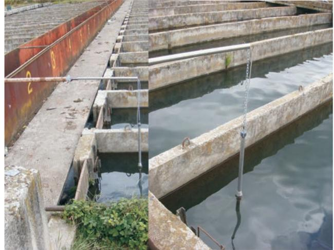
**Figure 2.** Mounting of the process probe for dissolved oxygen in the water outgoing from fish basin
