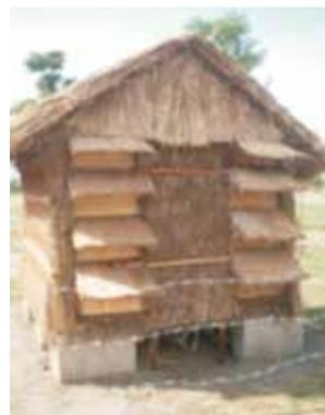
**Figure 2.** Improved Naturally Ventilated Storage Structure (INVSS)
